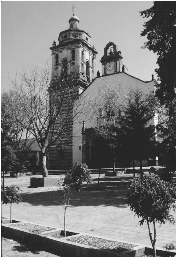
Plate 2 Church at Zinapécuaro, Michoacán. The obsidian-faced bell tower is on the left, and obsidian-chip designs set in concrete can be seen in the foreground (photo author).
