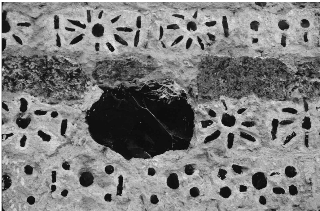
Plate 3 Detail of the bell tower at Zinapécuaro, Michoacán, showing a block of obsidian flanked by 'flower' or 'sun' designs composed of obsidian disks and fragments (photo author).
